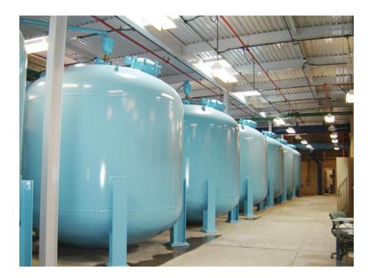
Figure 9. Pressurized Filters for Large-Quantity Treatment
