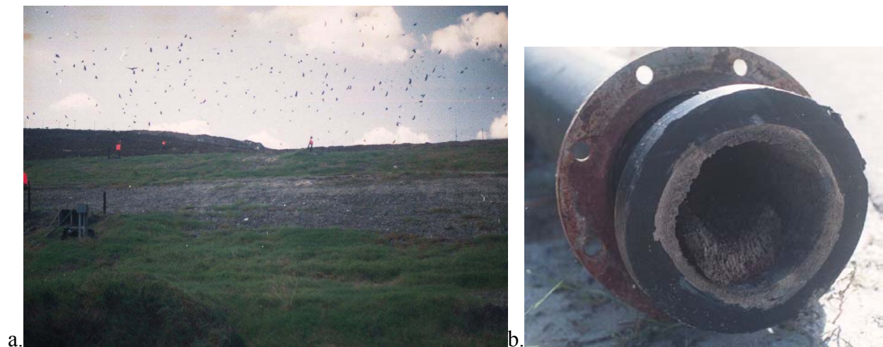
Figure 7. Southeast Florida landfill and clogged 8 inch pipe removed from leachate collection system.
