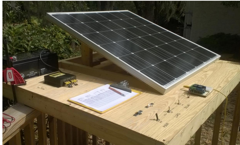
Power System Assembly
